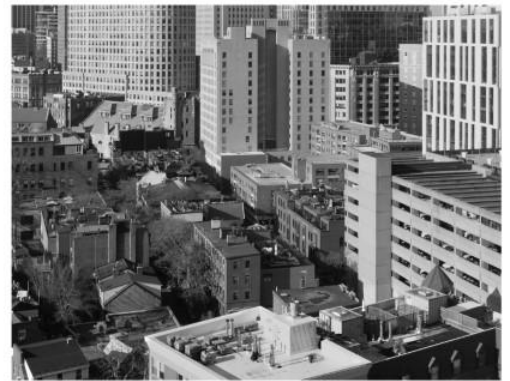
New views, aligned, Nov 2021 © Steve Dunwell
